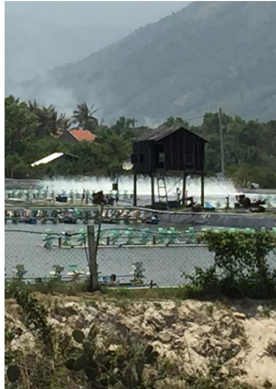
Smaller lined ponds with high levels of aeration
